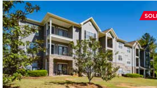
Stonegate Birmingham, Alabama 260 Units // Built 2008
