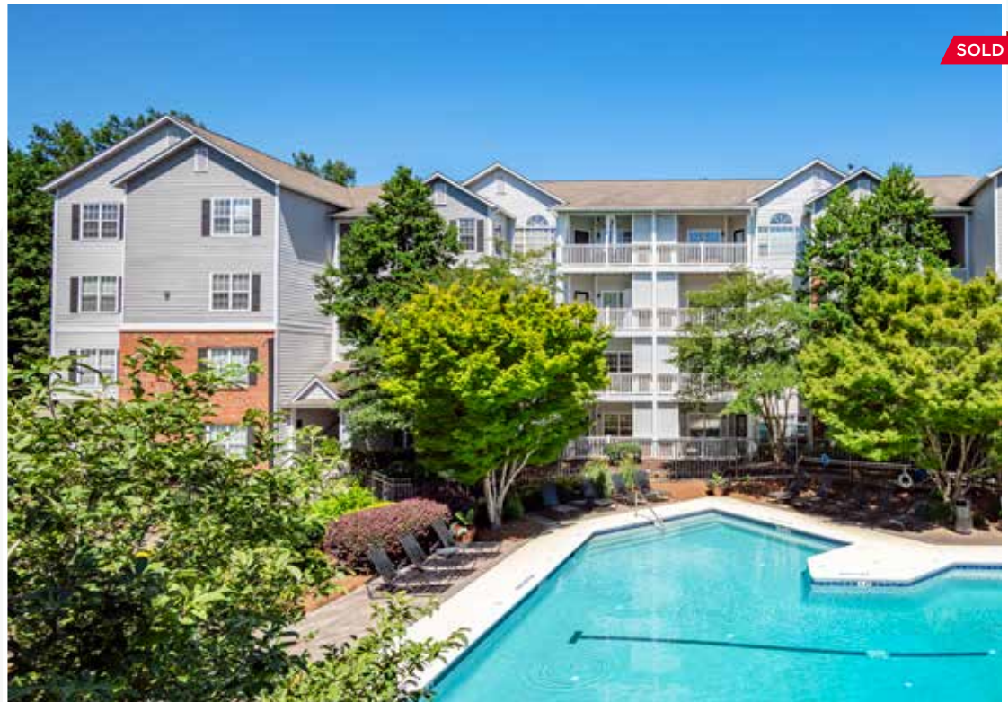
Aspire Perimeter Atlanta, Georgia 296 Units // Built 1996
