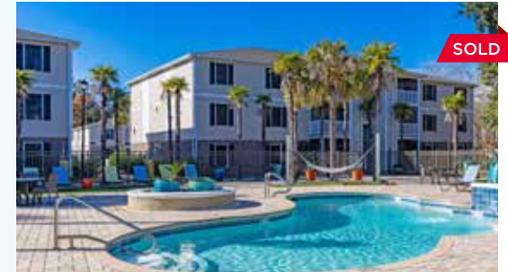
Grande View Biloxi, Mississippi 240 Units // Built 2003
