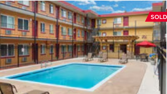
Newport Square Colorado Springs, CO 118 Units // Built 1973
