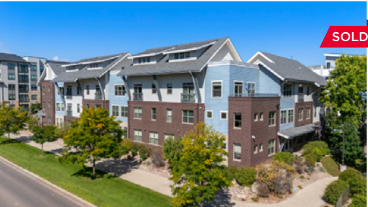
Apex & Haven Fort Collins, CO 113 Units //
